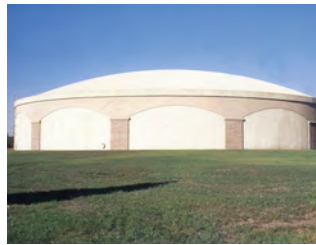
Above Ground Storage Tanks
