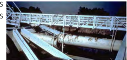
Damaged clarifier
